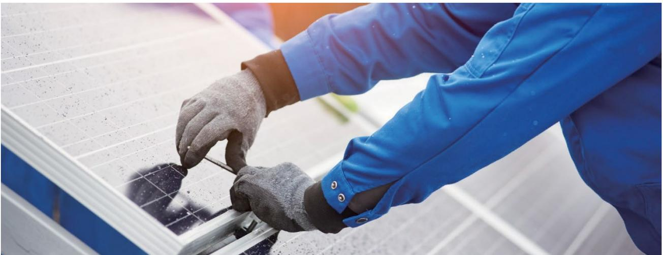
In extreme weather conditions or user-defined installation methods, strengthen key connections to prevent damage to modules or system connections.
